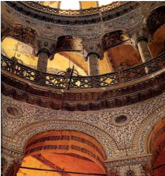
Fig. 6. Hagia Sophia, intercolumniation vaults, semicircular gallery, southwest corner)
